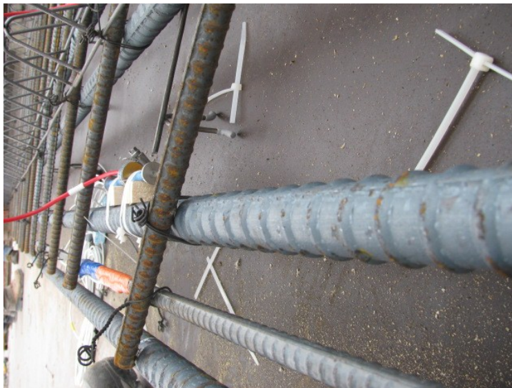
Figure 3.21: ERSG and VWSG placement – side view (typical)
