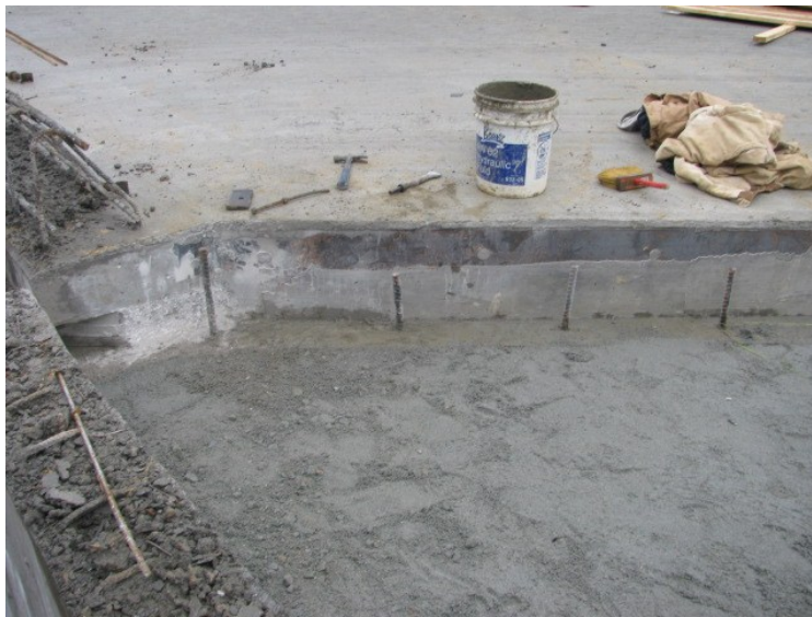
Figure 3.3: Cast-in-place bridge deck ledger
