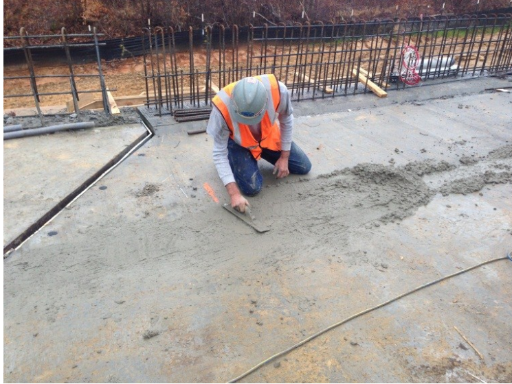
Figure 3.30: Shear key closure being finished
