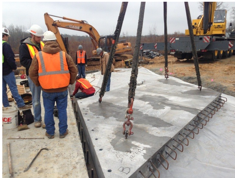
Figure 3.5: Interior approach slab being set with vertical dowel alignment
