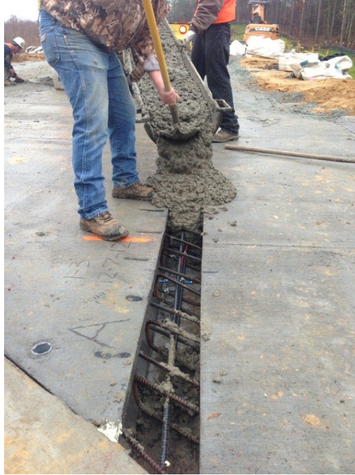
Figure 3.28: Placement of concrete in an instrumented shear key closure
