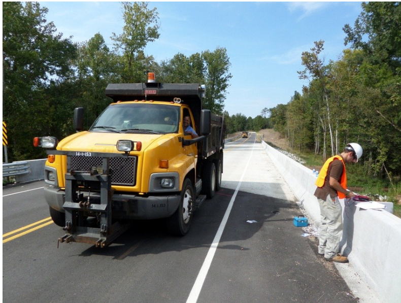
Figure 3.43: Static load testing: Load Case 3
