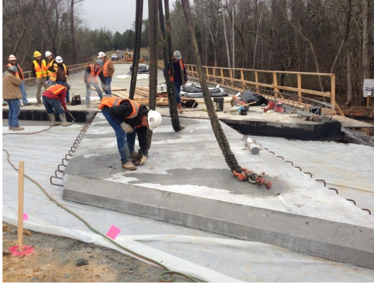
Figure 3.23: Placement of interior slab 'C'
