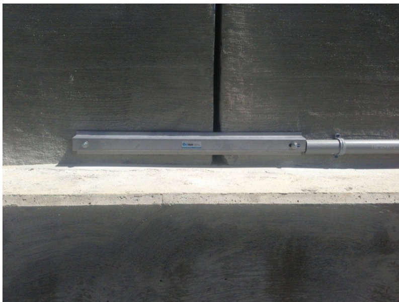
Figure 3.34: Installed cover plate (typical)
