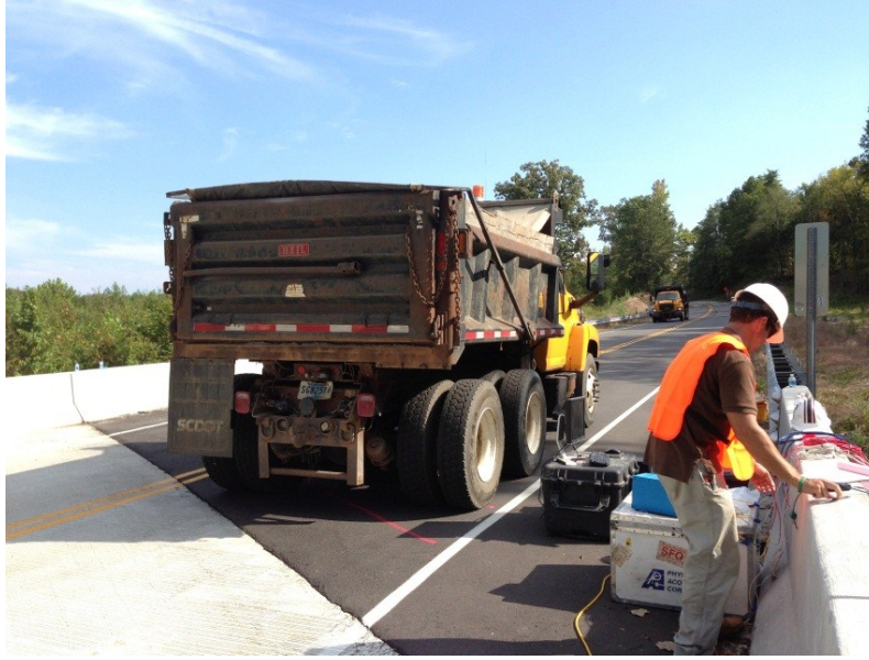
Figure 3.44: Static load testing: Load Case 4
