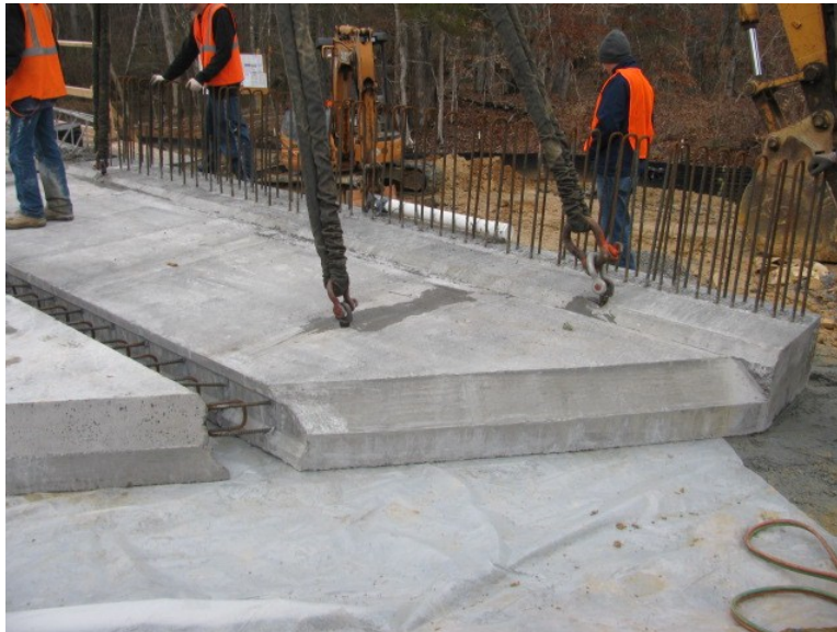
Figure 3.24: Placement of exterior slab 'D'
