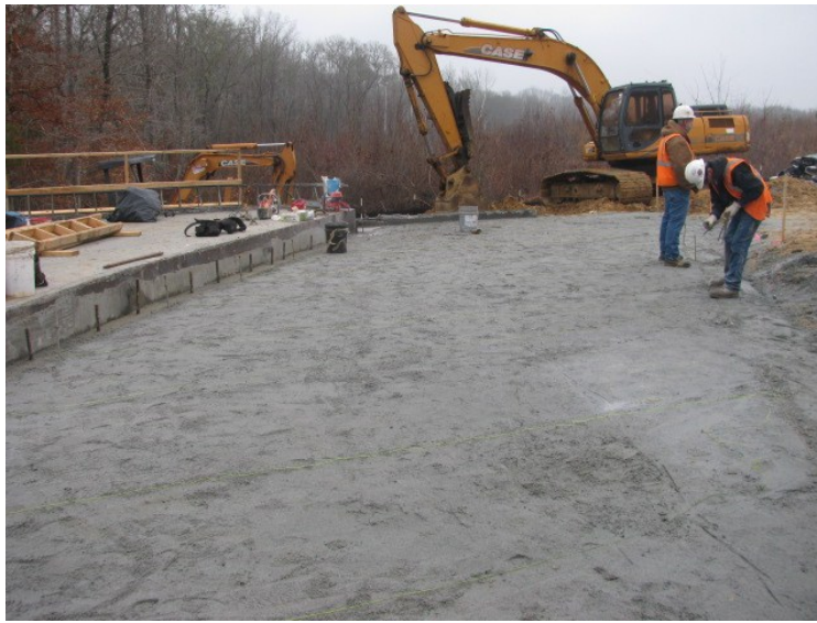
Figure 3.2: Compacted crushed stone sub-base material on the Bent One approach
