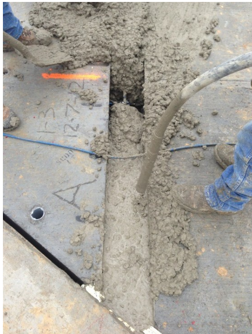
Figure 3.29: Concrete being vibrated during placement
