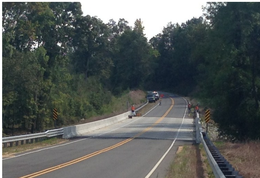
Figure 3.9: The completed replacement bridge over Big Brown Creek
