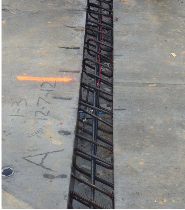
Figure 2.2: Improved connection shear key joint detail
