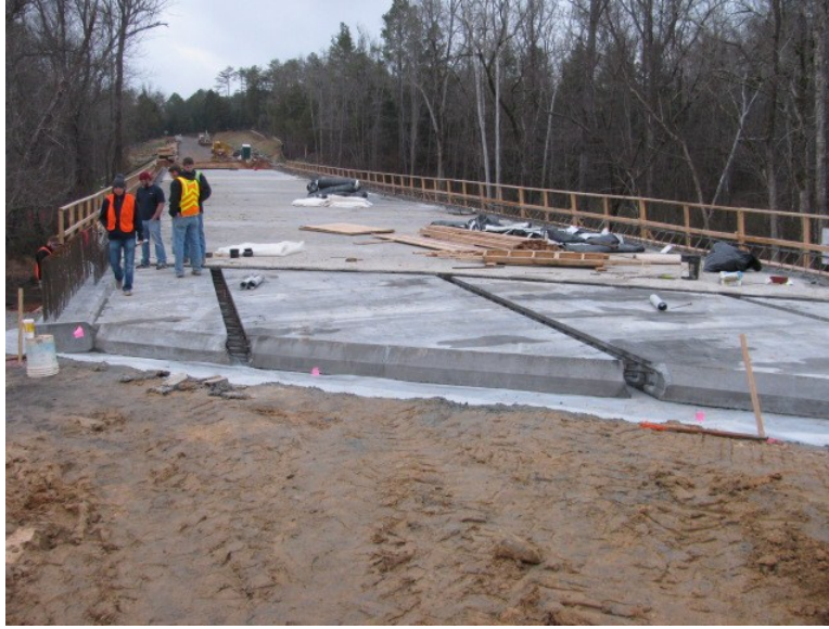
Figure 3.25: All approach slabs in place
