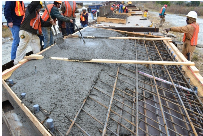
Figure 3.22: Concrete placement - interior slab 'B'
